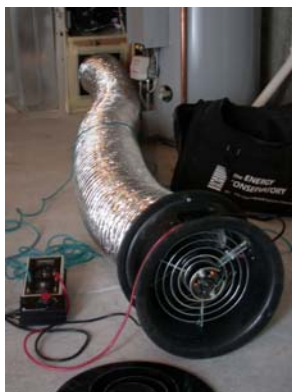
Total Duct leakage
